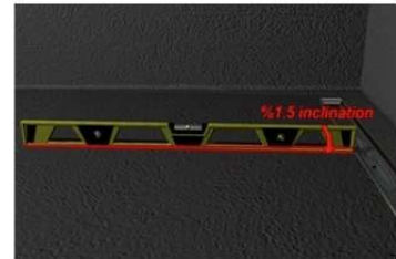
Doing the necessary beveling before ground cladding
