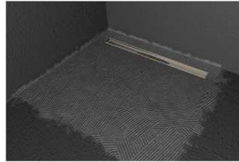
Glue implementation before ground cladding
