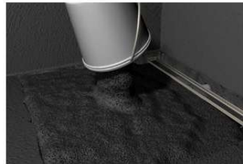
The applied cement finish will be kept lacking depending on the thickness of the ground cladding material
